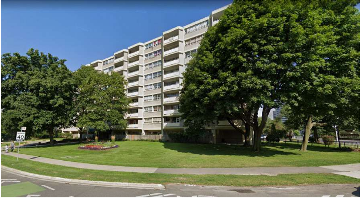
South East Corner along Grenoble Drive – Facing North West
